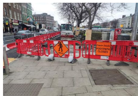
Works commencing on Burgh Quay
